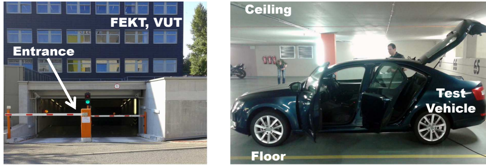
Figure 2: [left] Underground garage where the measurements were conducted. [right] Test vehicle and its surroundings.
